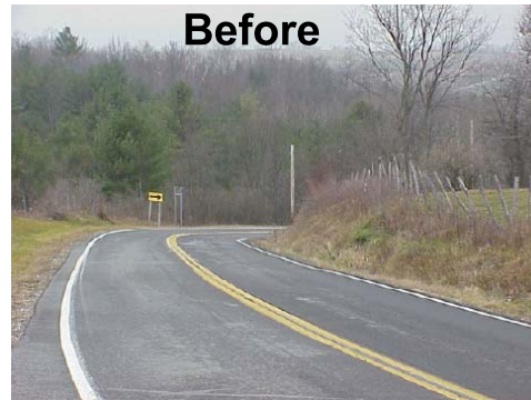
Poor visibility and clear zone issues
