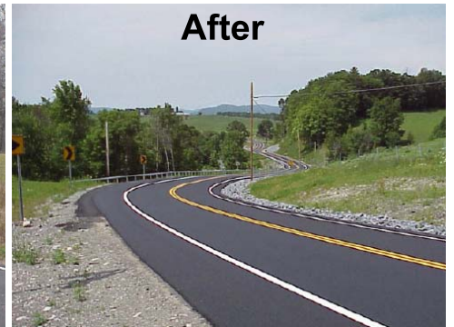
Roadside & visibility improvements; guardrail and delineation improved
